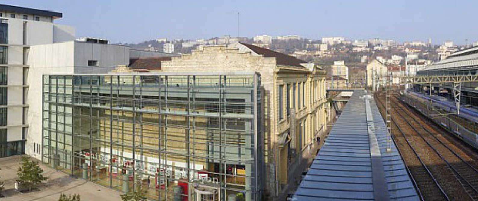
Work is in progress to simplify pedestrian and bike routes through the multimodal hub
