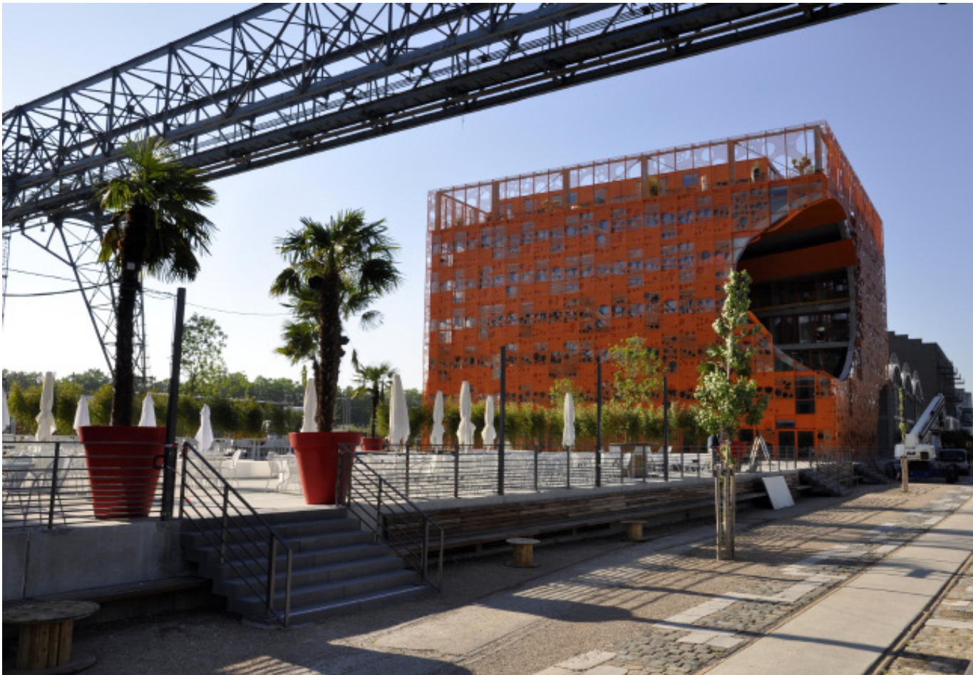
“Le Cube Orange” by architects Jakob + Macfarlane, home to the HQ of construction group Cardinal
