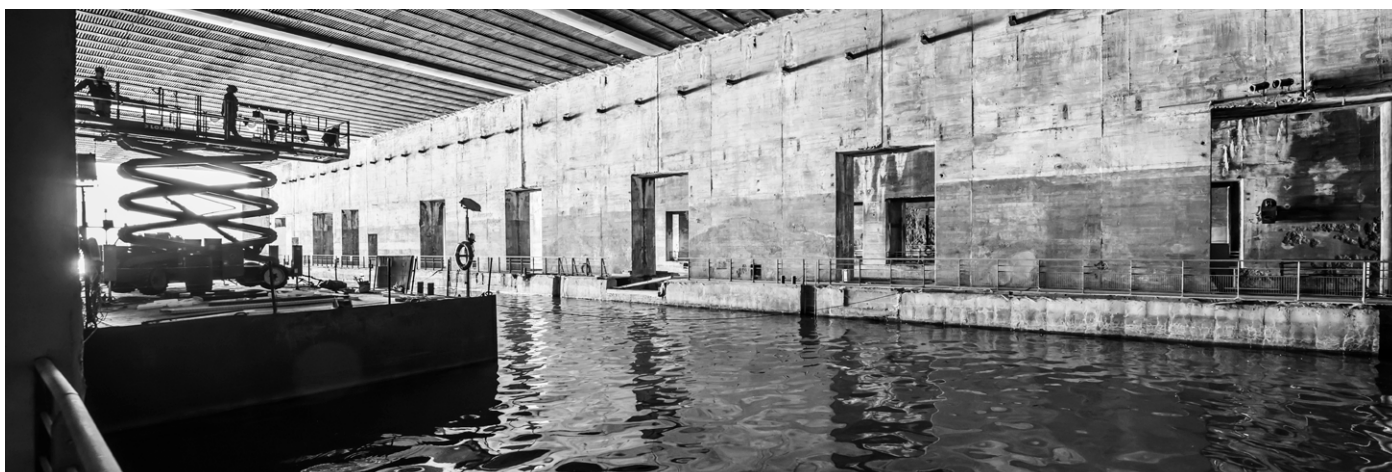
Restoration work – the Bassins de Lumières
